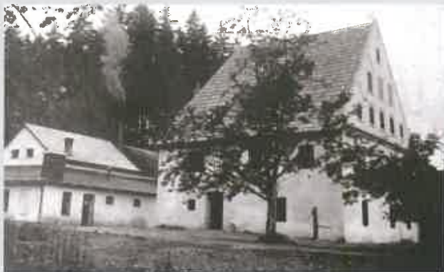
Power plant building and paper mill administration building (right) in 1915. The tall shingle roof with the attic space of the administrative building was originally used for drying sheets of paper, the National Heritage Institute, the photographic collection of the State chateau Hradec nad Moravicí
